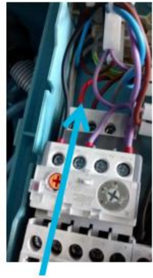
Non-modular units: disconnect red output cable to compressor contactor.
