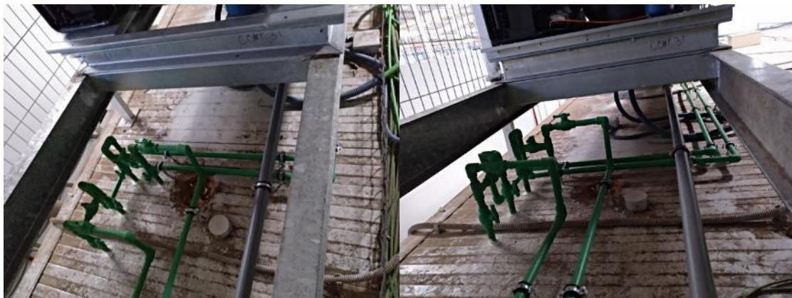
Mounting pipes with bypass in covered shed
